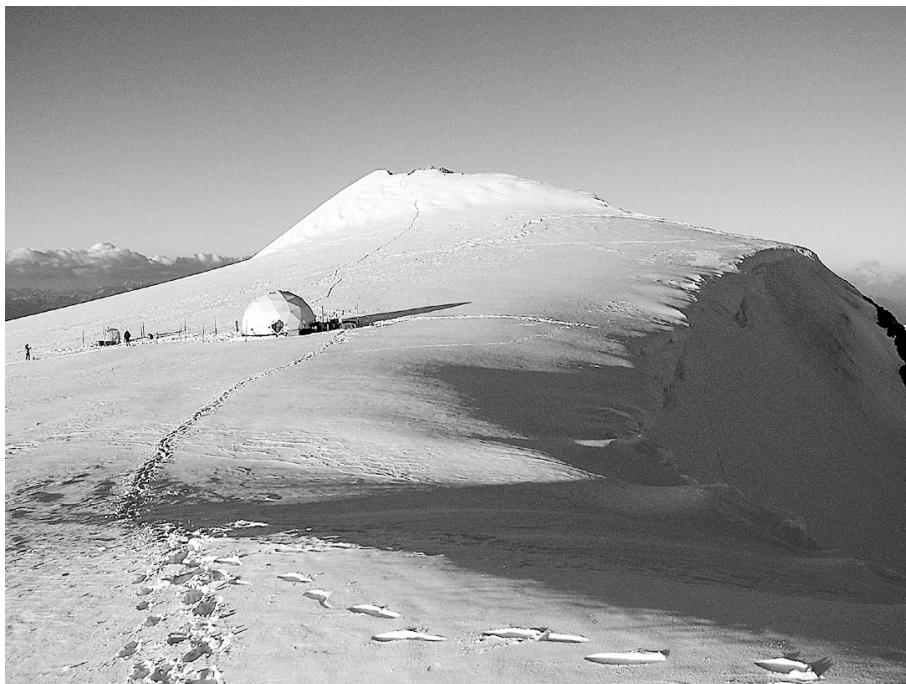
FIG. 2 - The drilling dome built at 3859 m near the summit of Mt. Ortles (3905 m) (Photo by Paolo Gabrielli).
